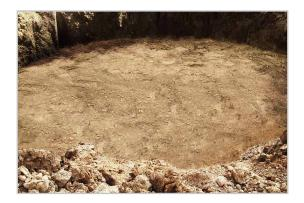
**1.** Remove all large and sharp stones or other hard objects from the pit, and create a bedding layer (at least 10 cm thick) of coarse sand.
