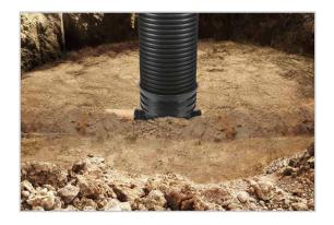
**4.** Clean the chamber base unit. Apply a lubricant to the inside of the chamber base unit and the seal on the rising pipe. Install the rising pipe securely, with the seal towards the chamber base units. The inspection chamber is ready to be buried in easily compactable soil. Bury the inspection chamber in layers, each up to 30 cm deep.
