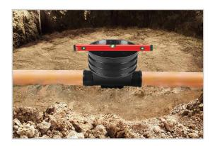
2. Position the chamber base unit on the sand bedding (remember to level it properly and consider the base unit base slope of 1.5%), connect the drainage pipes, and bury the chamber base unit to approximately 10 cm above the pipe height to secure the base unit against shifting.
